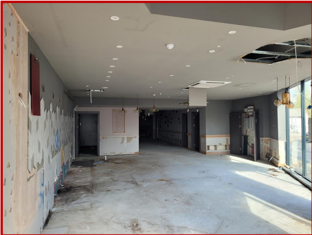
Internal photos of ex Costa – 723a
